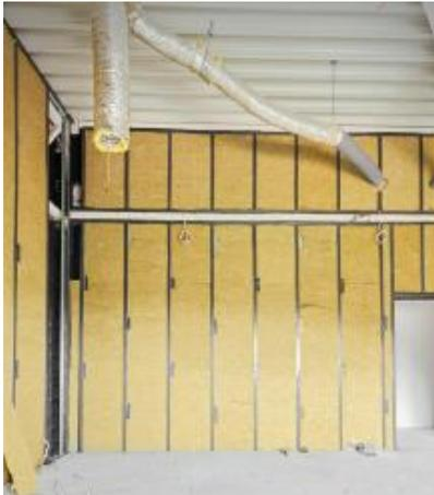
Figure 5018.3 Example of Continuous Insulation<sup>4</sup>
