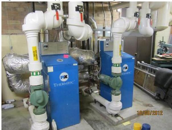
Figure 6005.6 Typical Steam Boiler
